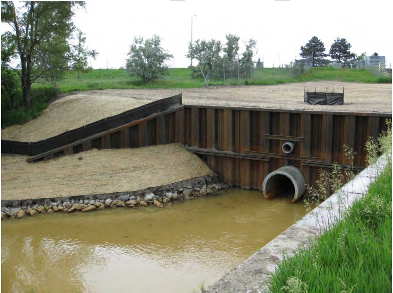
Example of sheetpile headwall with steel bracing
