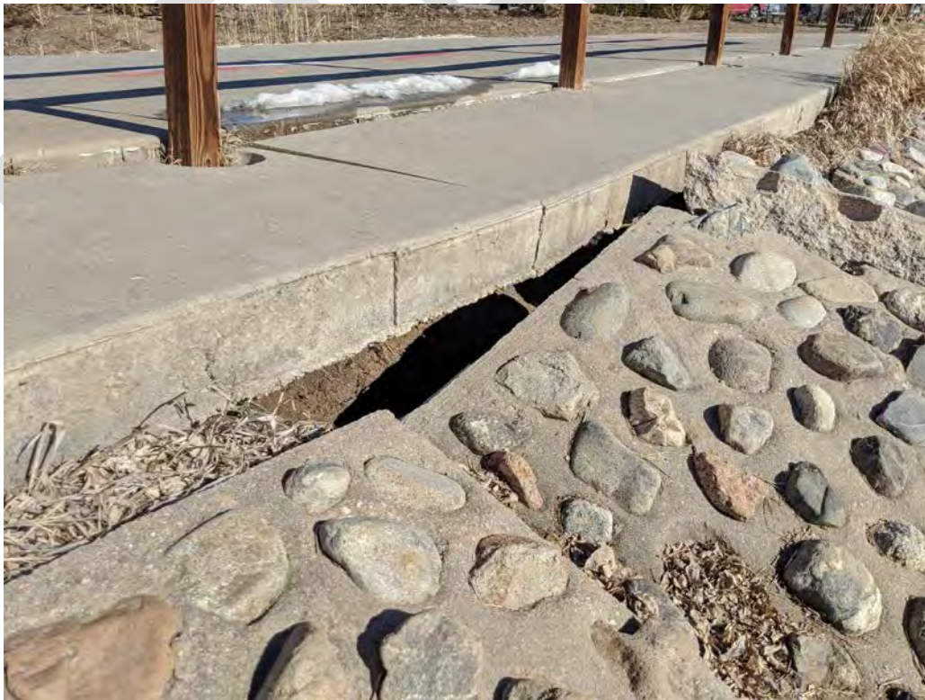
Undermining of slab adjacent to trail, handrails that will need to be reset or replaced
