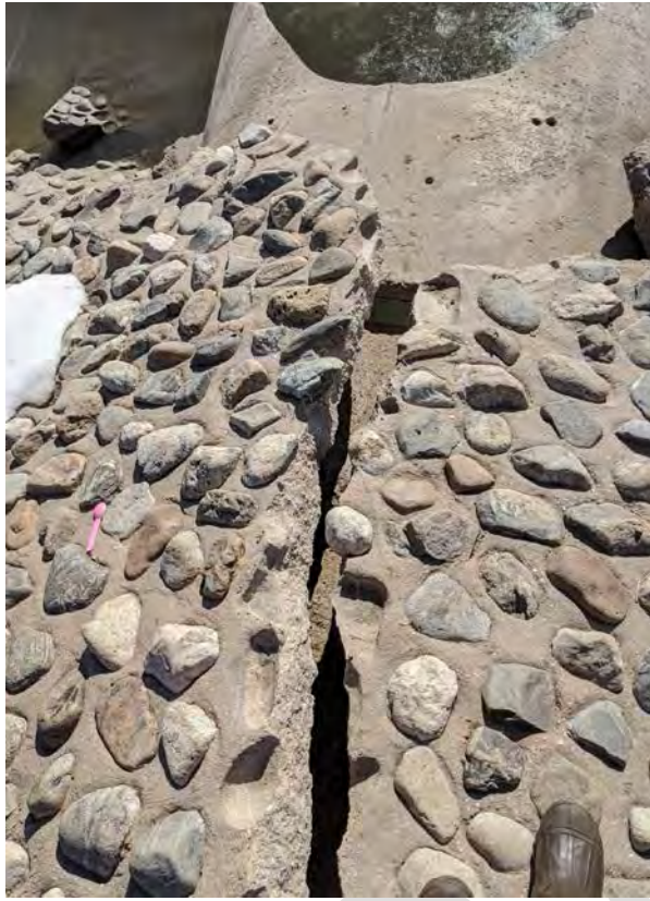
Grouted riprap cracking above the culvert
