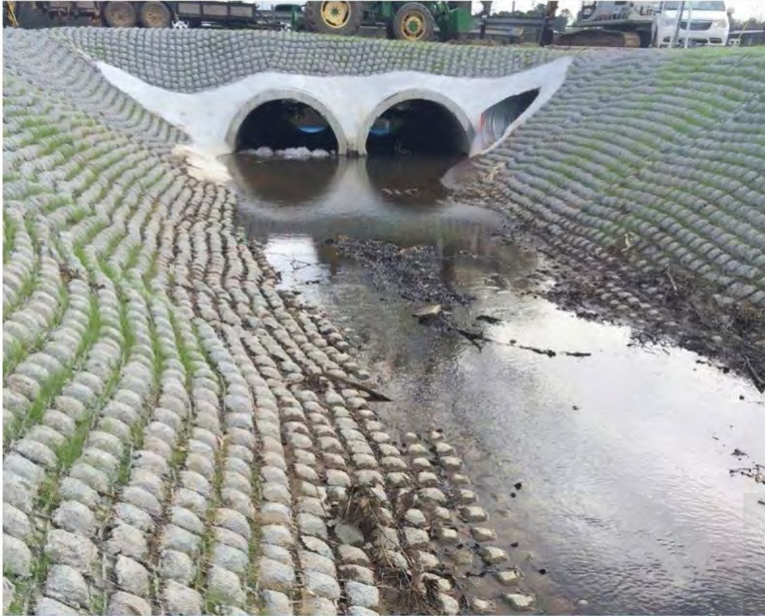
Example Flexamat used to stabilize an outfall and embankment with grout around outfall
