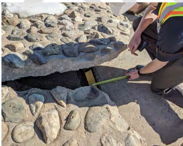
FES separation from culvert from the outside
