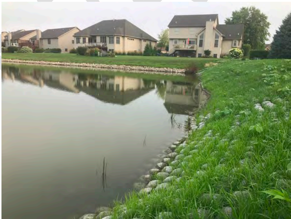
Example of Flexamat used around a lakeshore
